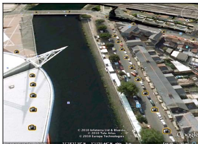
Aerial view of Riverside Market showing the edge of the Millennium Stadium
